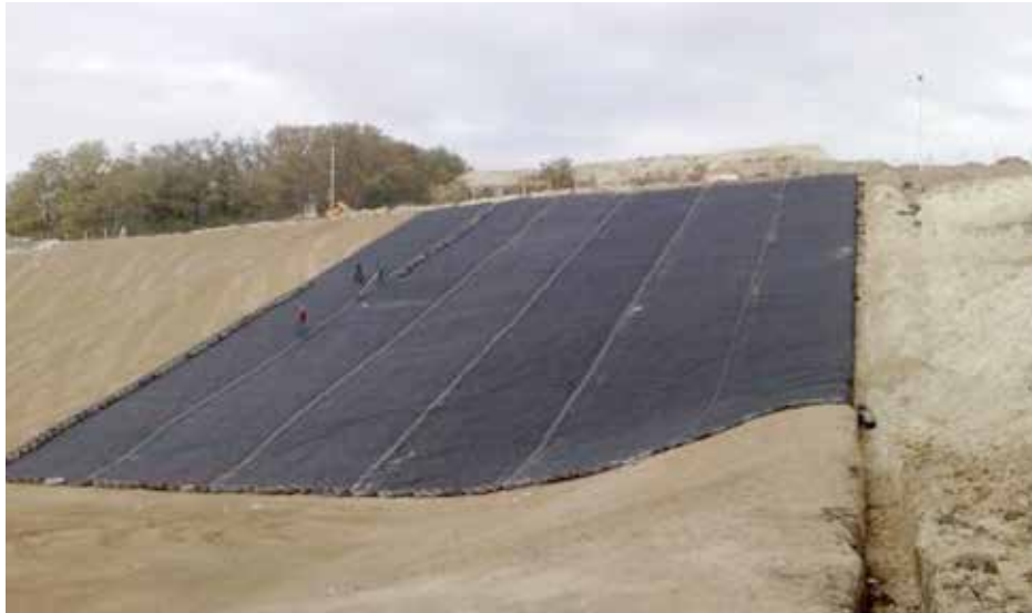
Fig. 35: Artificial barrier using HDPE foil for landfill
