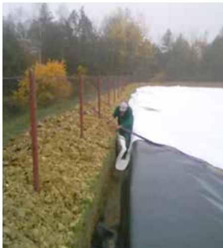
Fig. 36: Foundation of landfill
