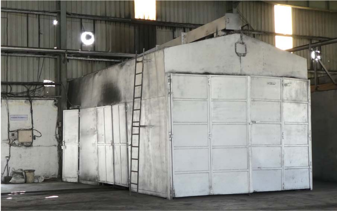
Encapsulated Centre Tapping Furnace ( Courtesy of Gravita India )
