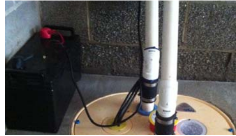
Capture Any Acid Spillage
