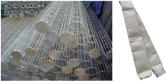
Typically Filter Bags Capture Dust to 25 microns ila
