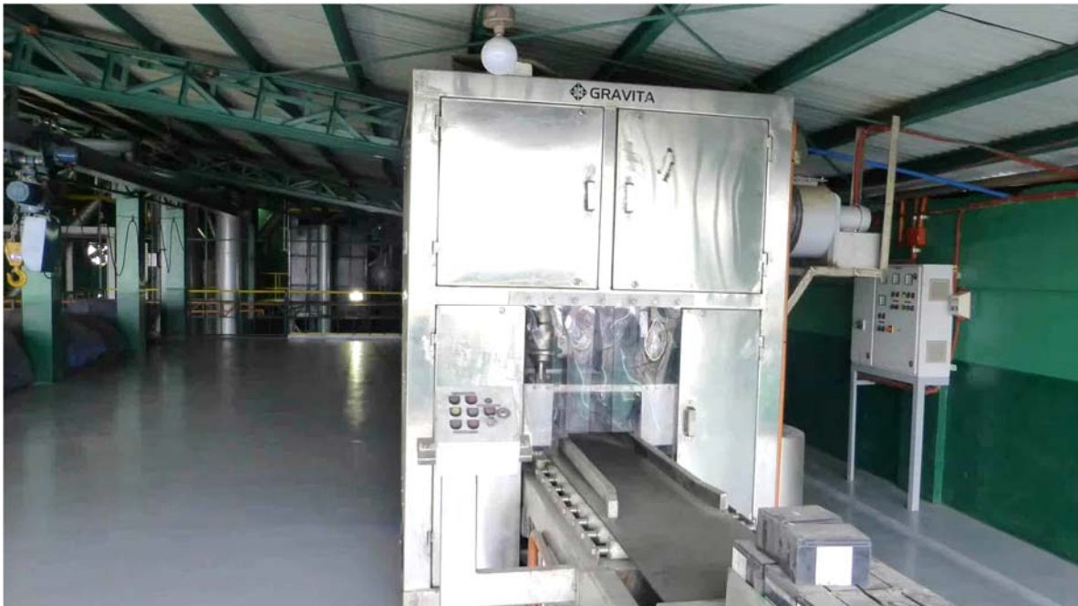
Ventilated Battery Saw ( Courtesy of Gravita India and Eco Global )
